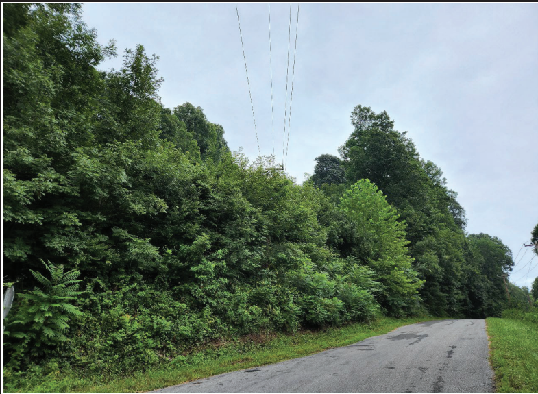
P-5b 44PK0049 View towards site and line
