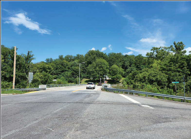
P-10c 044-5173 / NR-08000072 - Fieldale Historic District View of district
