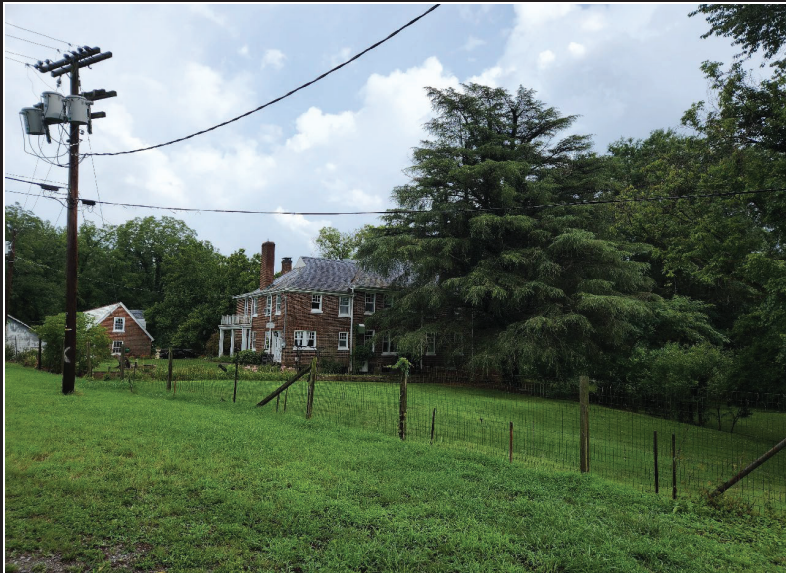
P-23c 044-5174 / NR-06000708 – R. L. Stone House View towards line
