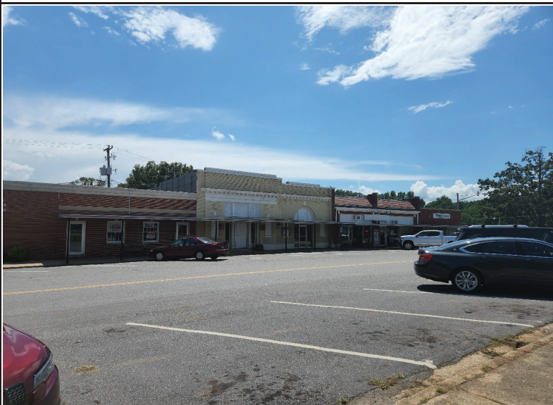
P-8a 044-5173 / NR-08000072 - Fieldale Historic District Towards Marshall street
